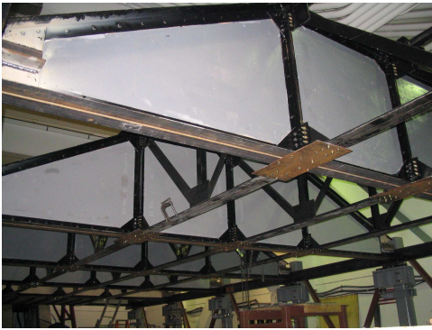
Figure 14: The Ceiling Structure
