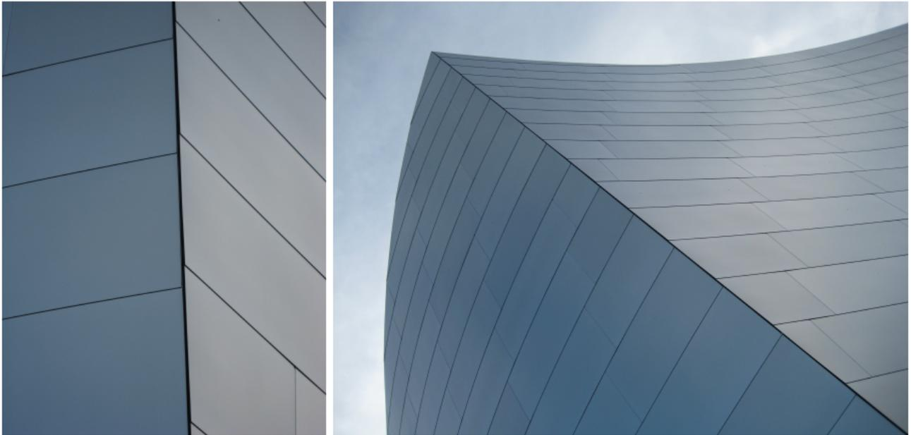
Assembling developable surfaces at a common crease leads to the **tiling problem** if the crease is not developable.
